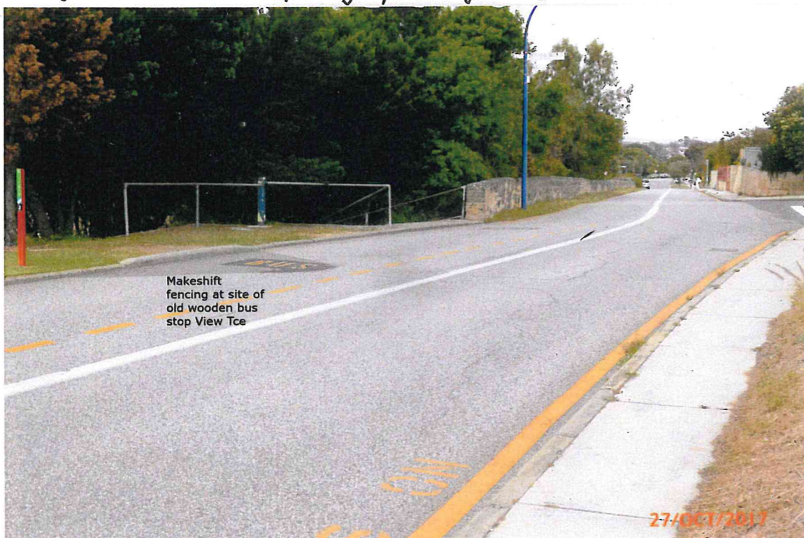
The end of the limestone wall near blue Street Post needs a reflective end point - hard to see in winter & night time
