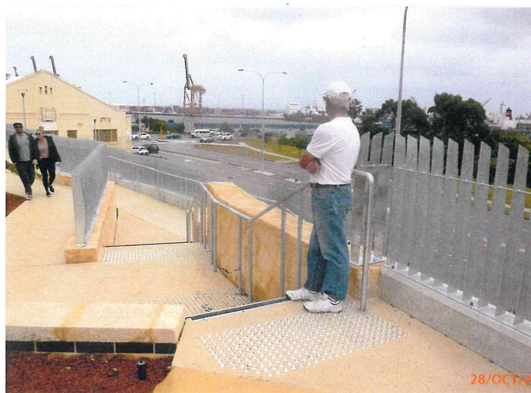
← Stairs from Tuckfield Oval Parkland, Fremantle leading down to Canning Hwy near Old Traffic Bridge with all the safety features NB The high, metal, blade, palisade fences for safety so kids (and adults!) can't climb over them. Similar palisades could be used around a future viewing platform in View Terrace.
