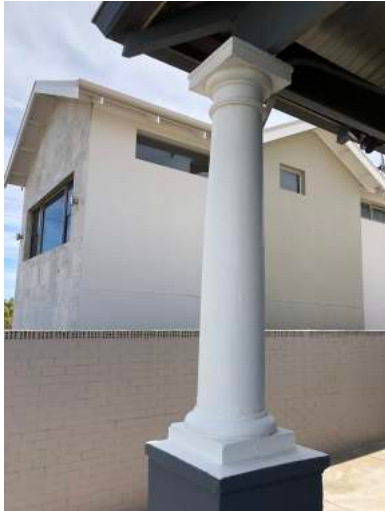
typical front verandah column to be replicated in re-instatement of western verandah
