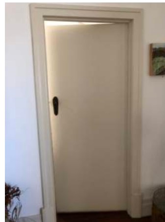
typical existing hollow core plywood internal door
