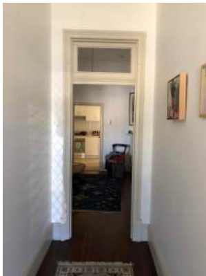
typical joinery to be retained including top light to front door
