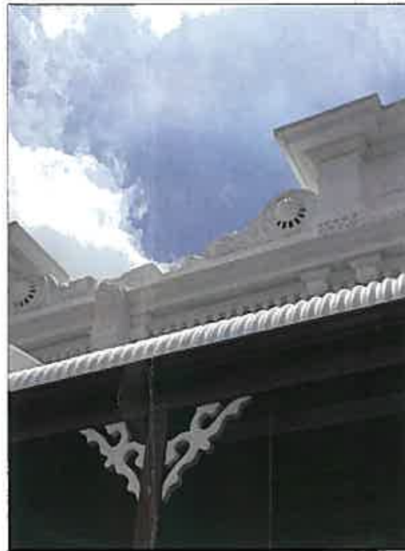
NOTE: TIMBER COLUMN & COLUMN BRACKET DETAIL AT NEIGHBOURING RESIDENCE
